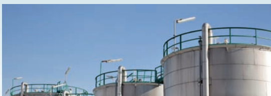
Tank Level and Temp Monitoring & Control
